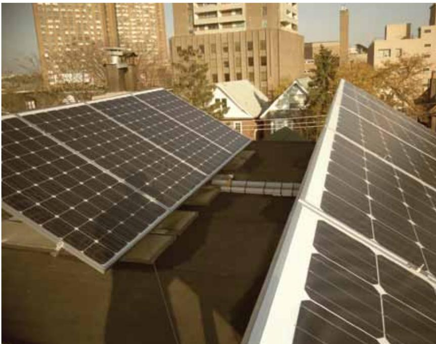
**Temperature plays a significant role in PV power production, according to Enphase Energy. As a general rule very 1°C increase in cell temperature will result in a 0.5% decrease in power. Clear cold weather is ideal for PV output. Here a 2.35kWh solar panel installation in Toronto.**
