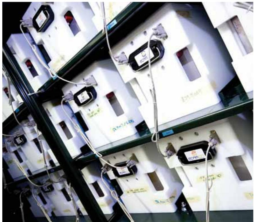
**Inside the box: an array of lithium batteries that can deliver 250kWh of storage**
